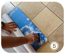
Line up the adhesive film on the plastic diffuser. Use the felt tip squeegee provided and slowly move from one end to the other removing all air bubbles.
